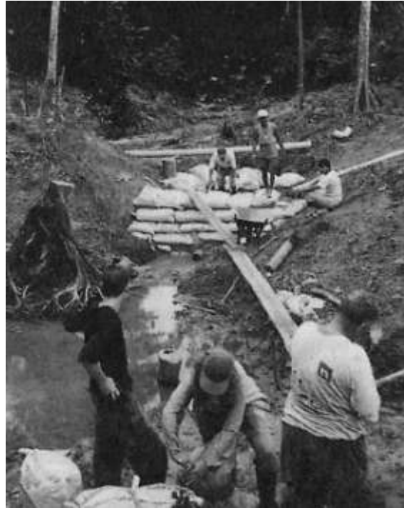
Dam building to create an artificial beach
