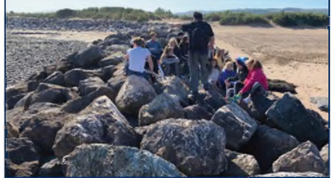
A group of Year 11s experiencing a rock armour groyne at Minehead and the resulting Terminal Groyne Syndrome.
