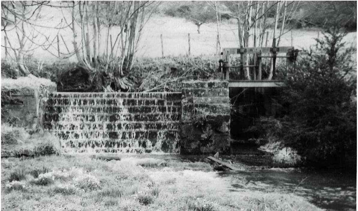
CHURN WEIR (CM Swaine's House) : 1973
